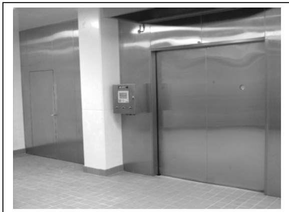
Horizontal sliding door autoclave installed @ site
