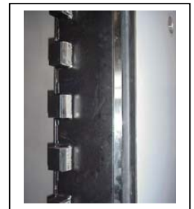
Door block & leading edge safety sensor
