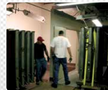
Continuing sequence showing sections navigating through corridors and rigged into their final destination.
