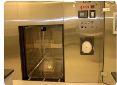
Vertical rising door autoclave installed at site.
